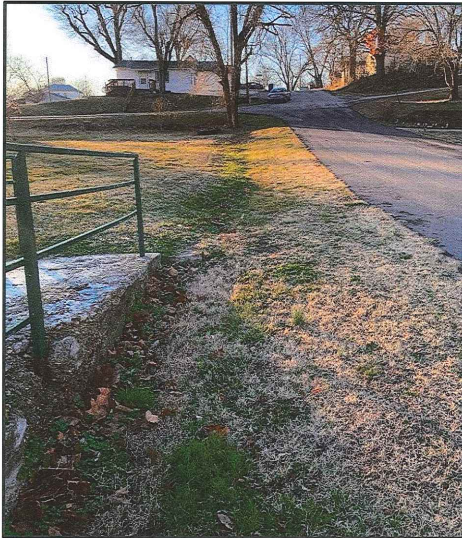
Figure 7: Ditch along Sixth Street with minimal capacity
