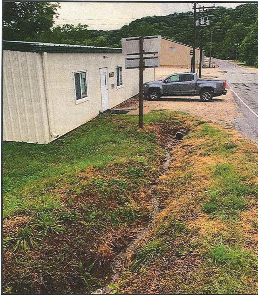
Figure 3: 12" CMP under Meta City Hall parking area along MO-133
