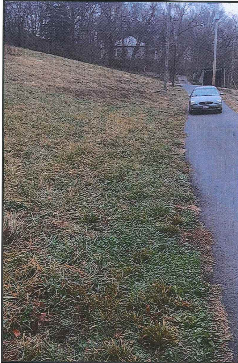
Figure 9: Lack of defined ditch along Schriefer Street
