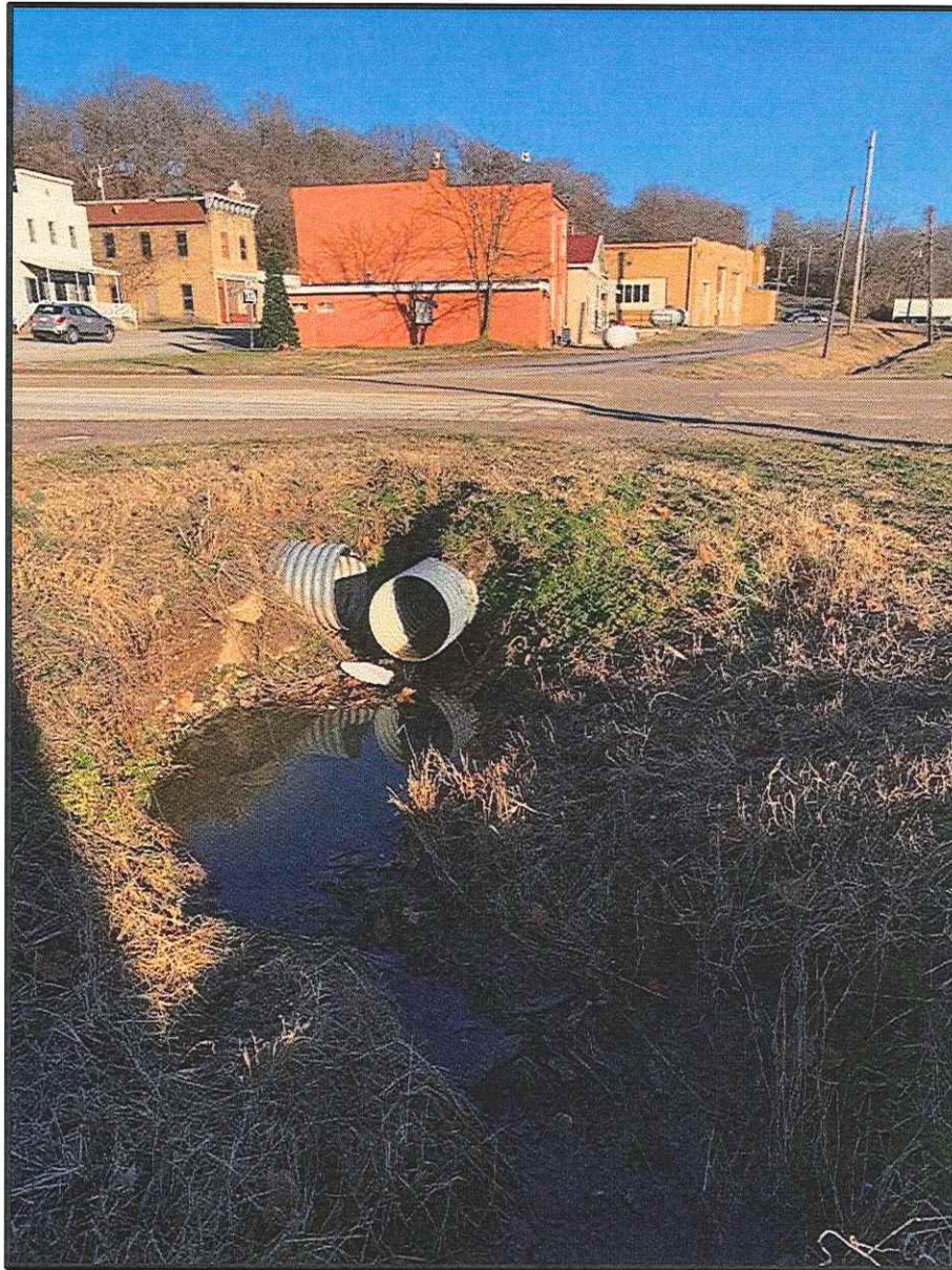
Figure 11: Perpendicular culverts intersecting at Bertha Street
